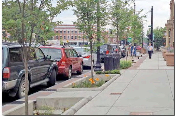
North Street, Pittsfield, MA. Bioretention Planters receive stormwater from the street and sidewalk. Photo courtesy of Vanasse Hagen Brustlin, Inc.
