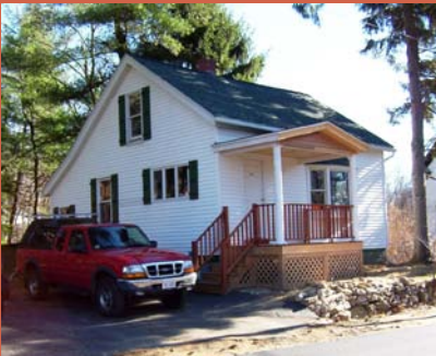
Figure 20: After photo. New porch, façade and roof.
