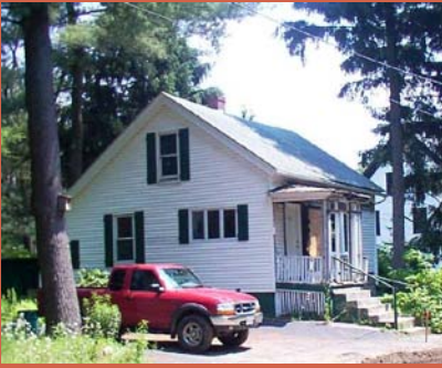
Figure 19: Before photo, home on Warren, MA. Dilapidated front porch, front façade, and roof.
