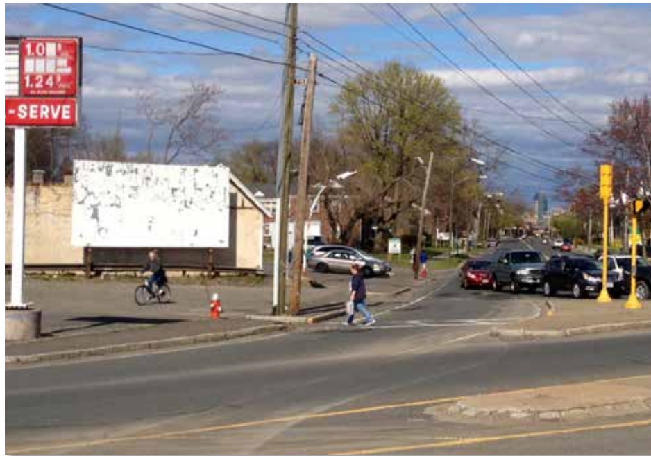
Poor crosswalks and numerous curb cuts degrade safety.
