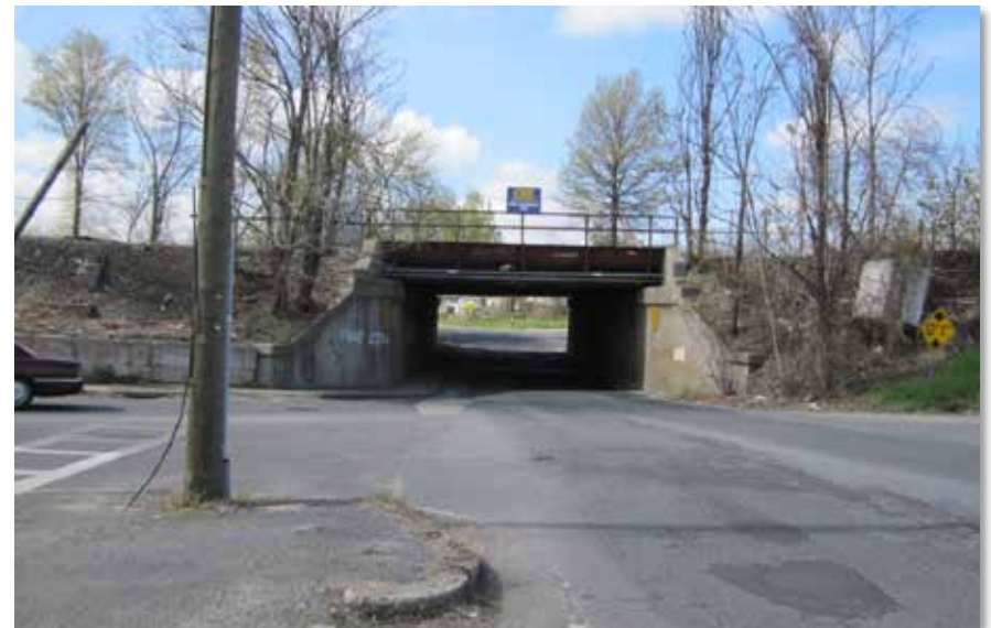
Union Street Underpass
