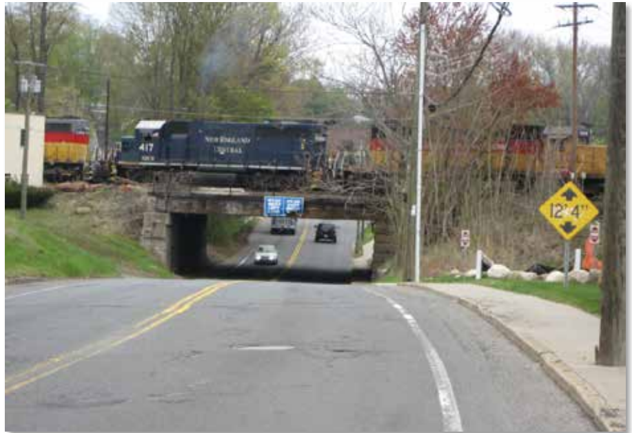
River Street Underpass
