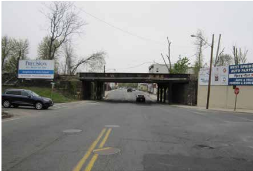
Main Street Underpass
