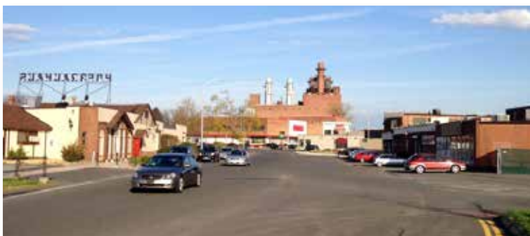
Existing Conditions. Lack of lane striping, curbs and crosswalks on Main Street are a safety concern for vehicles and pedestrians.
