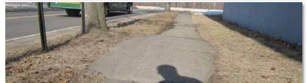
Existing sidewalks and school crosswalks are in poor condition.
