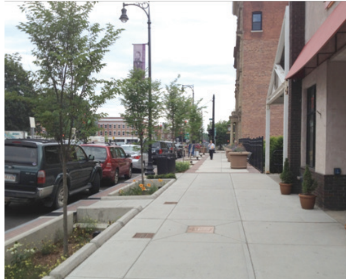
After: Street drains through curb cuts to bioretention planters.
