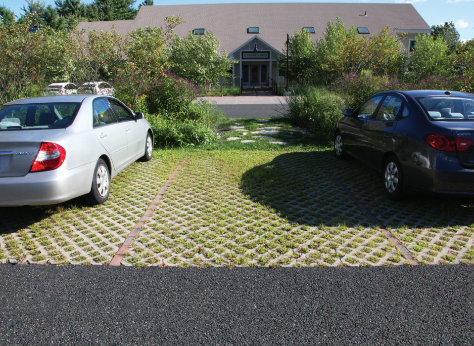
Rain gardens, porous pavers and asphalt are featured in this parking lot at New England Environmental, Amherst.
