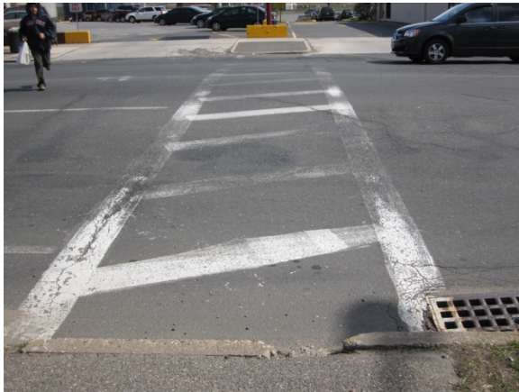
Non ADA compliant pedestrian crossing
