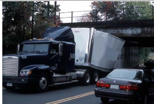
Truck stuck under a low clearance underpass in West Springfield
