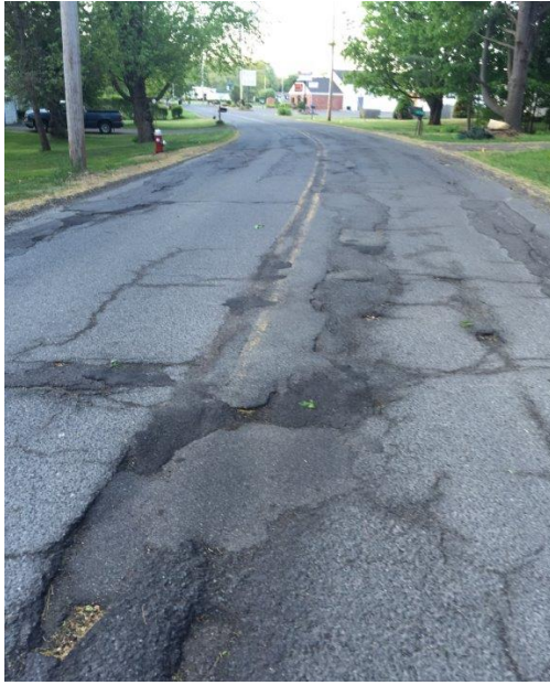
Poor pavement condition on East Street in South Hadley, MA.
