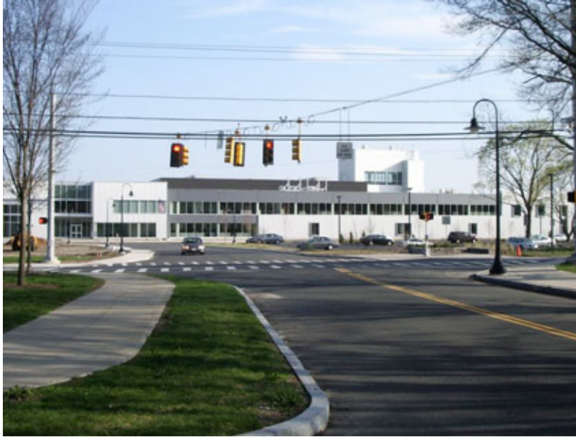
New Kollmorgen Electro-Optical Facility – Village Hill, Northampton Photo by Teri Anderson
