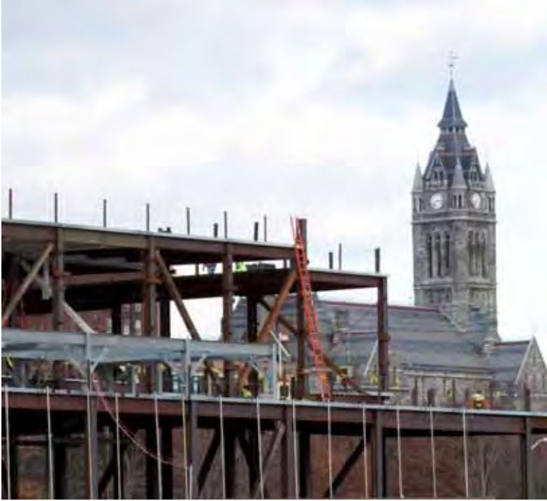
Massachusetts Green High Performance Computing Center under Construction with ca. 1874 Holyoke City Hall in Background Photo by Raphael Centeno
