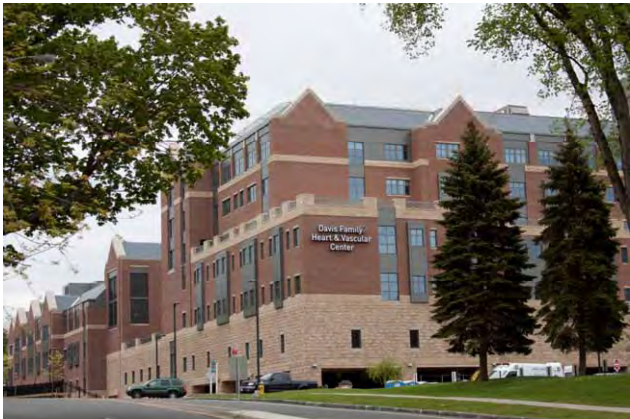
New MassMutual Wing with Davis Family Heart and Vascular Center at Baystate Medical Center, Springfield Photo by Raphael Centeno
