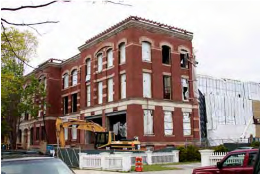
Redevelopment of Technical High School as State Data Center in Downtown Springfield Photo by Raphael Centeno
