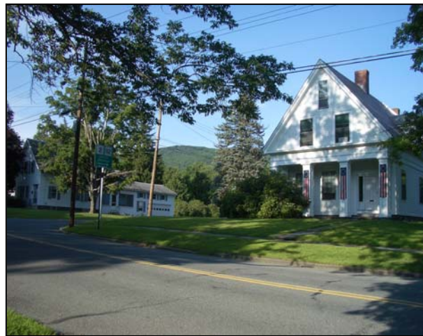
Intersection of Hope and Main Streets, Shelburne
