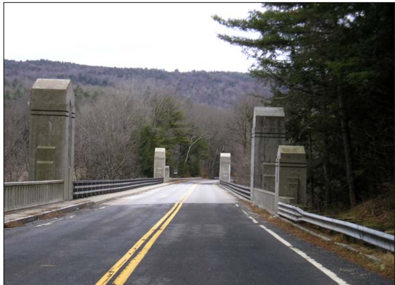
Route 112 crosses the East Branch of the Westfield River in Huntington
