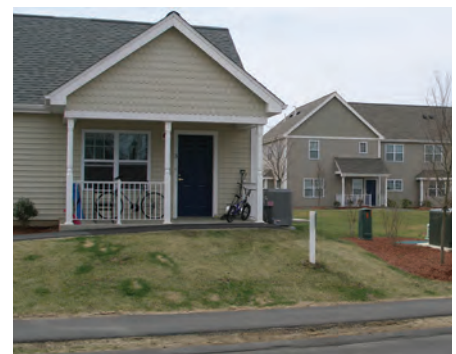
Home with barrier free entry at Tree House Development in Easthampton. Source: PVPC
